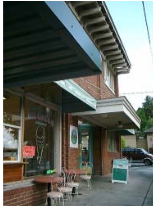
Canopies providing weather protection
