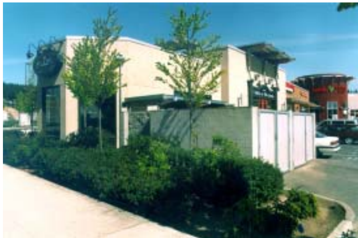
Dumpsters screened by walls and planting strip along sidewalk
